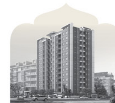
Suraj Height Jaipur (September 2022 - March 2024) Residential Project
